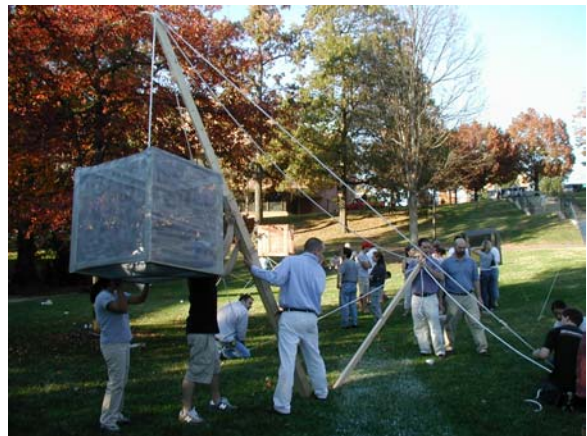
Figures 11a & b. Cube project at desktop model scale and full-scale erection.
